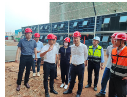
On-site Inspection of the Hainan ITG Smart Logistics Park Project
